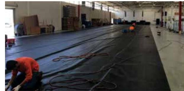
**PHOTO D** Fabrication—Detail work and capping cross-seams.
